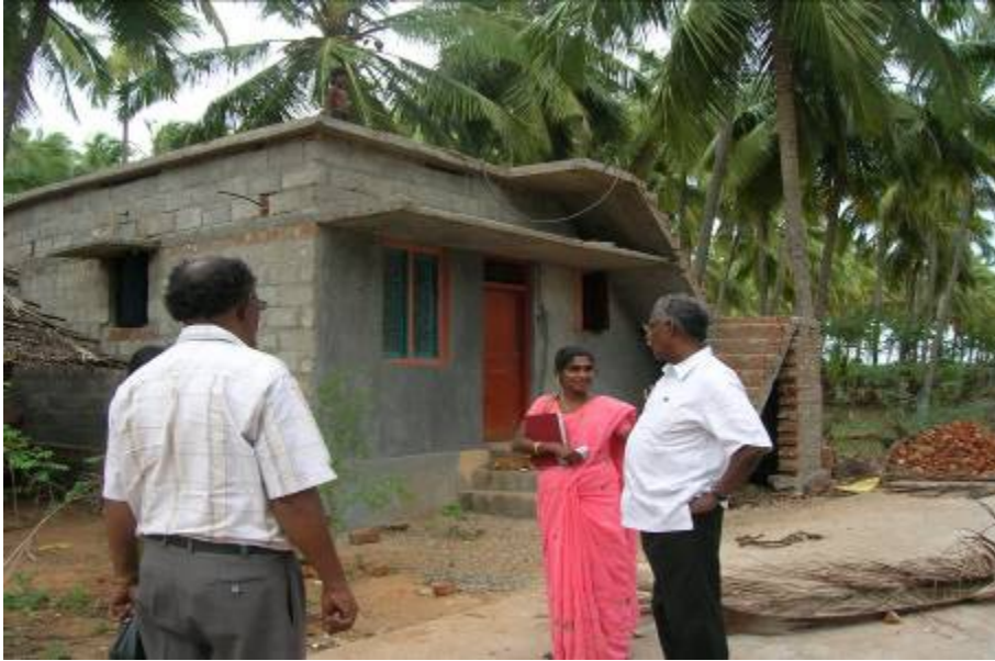
Completed house with habitat funds and locally available materials.
