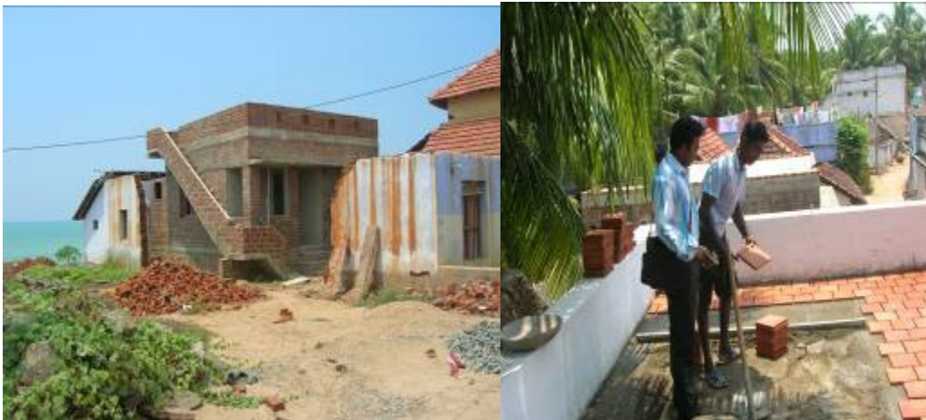
Houses under construction in RGRP programme.
